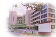
St. Marks Hospital
